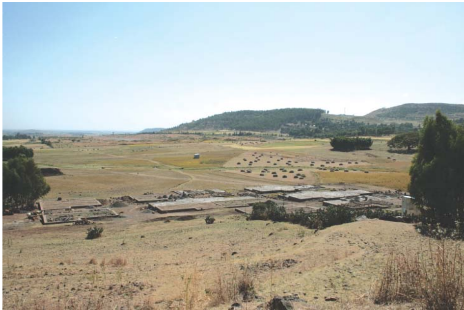
FIGURE 10 New buildings at the limits of Azazo. Jaime Almansa.
